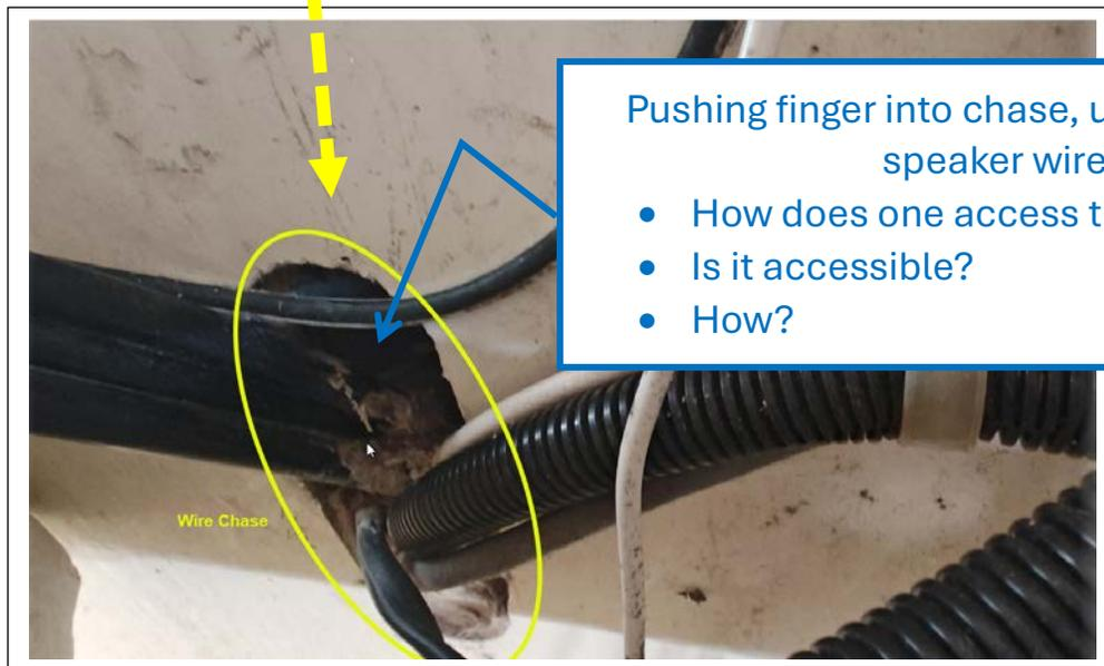
Pushing finger into chase, unlikely to pass speaker wire
